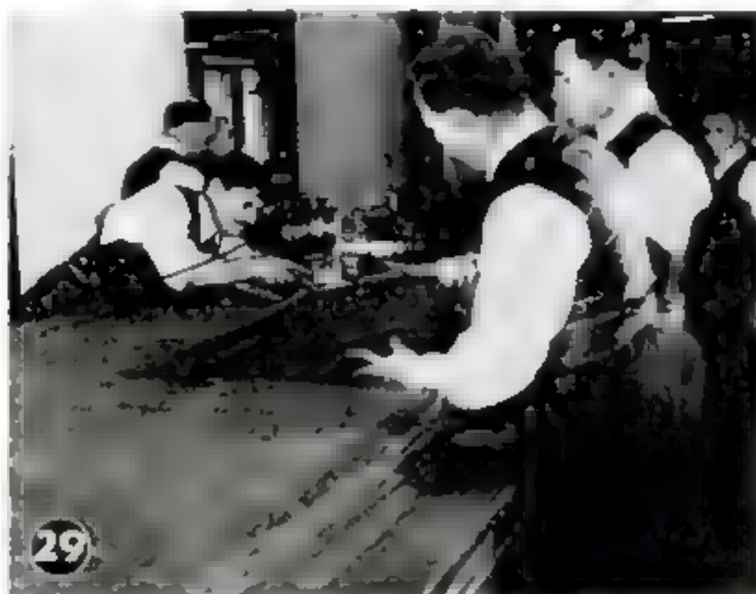
29 Making 14,000,000 uniforms for Army is speeded by this electric cutter which slashes into bolts of khaki, cuts 60 uniforms at once.
